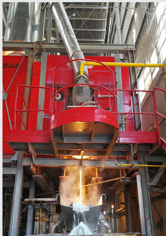
کوره ثابت Continues kiln
